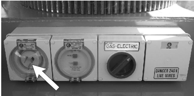
Figure 11.11 - AC Power Input Connector
